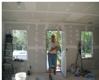
Allen Schramm working on drywall and closets in the new house.
